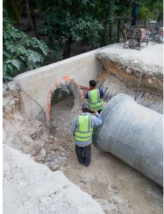
36 inches diameter culvert installation
