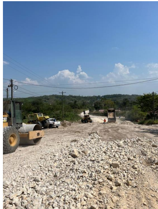
Road rehabilitation, dumping, grading, re-compacting
