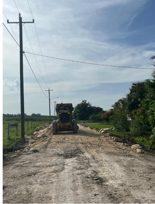
Spot dumping and grading
