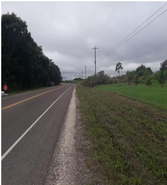
Mechanical Vegetation Control, Corozal
