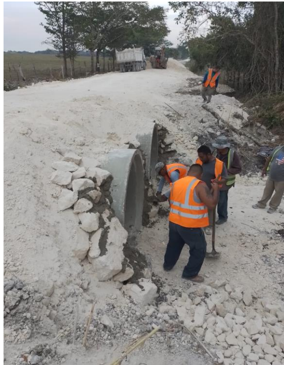
Preparation for end structure construction
