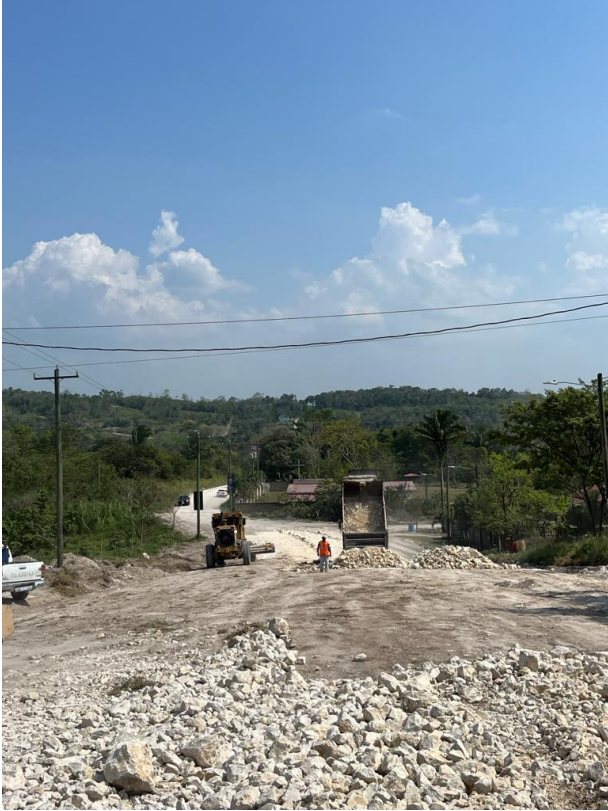
Street expansion – dumping pavement quality material
