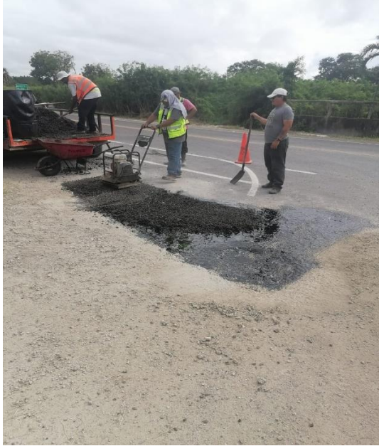
Pothole Patching with Pre-mix asphalt
