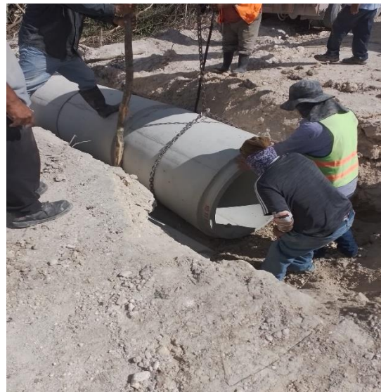
18 inches diameter RC pipe culver installation
