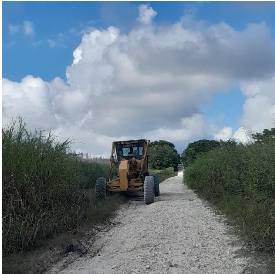
Drainage shaping with grader, Sugar road maintenance
