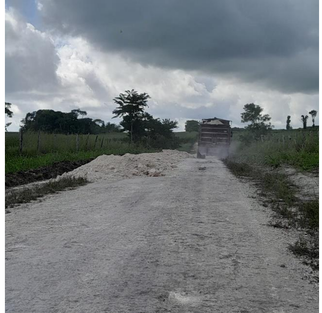
Spot Dumping and Grading with shoulder works
