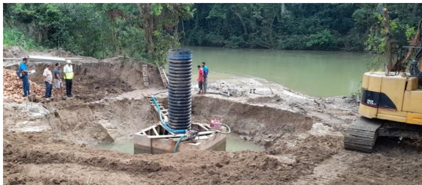
Fig. 25 Santa Familia RWS rehabilitated water gallery
