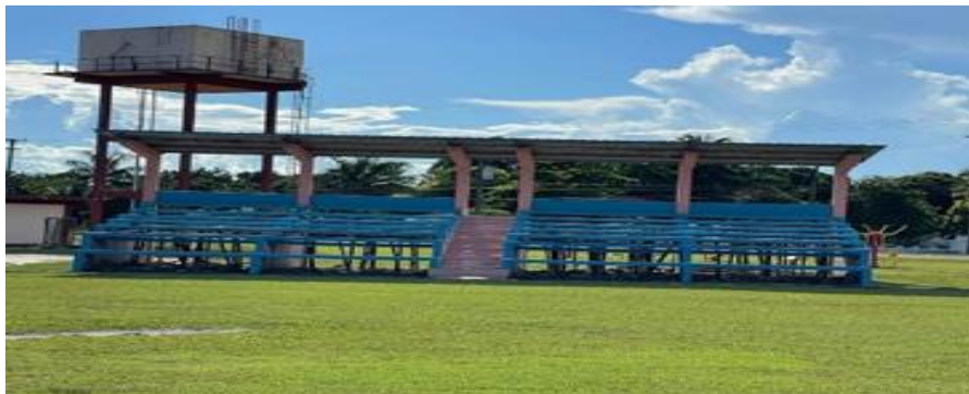
Fig. 21 Improvements to San Narciso Village Bleachers
