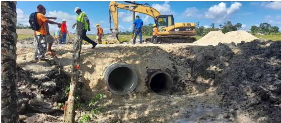
Fig. 17 Installation of culvert in Los Tambos
